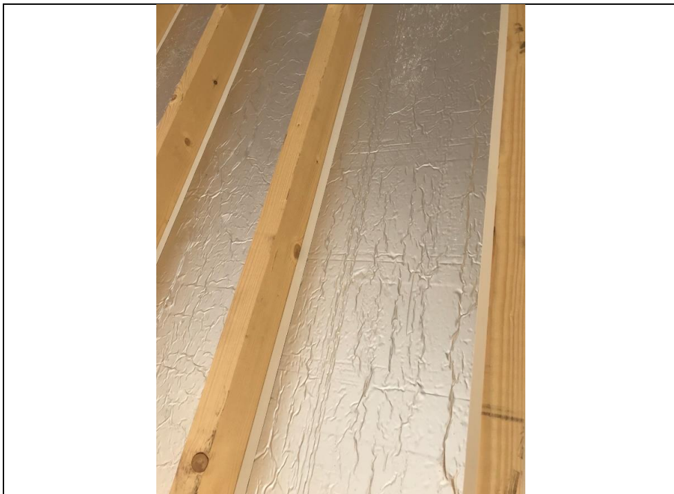
Figure 8 Insulfix Track – installation onto underside of rafters (new build - external view)
