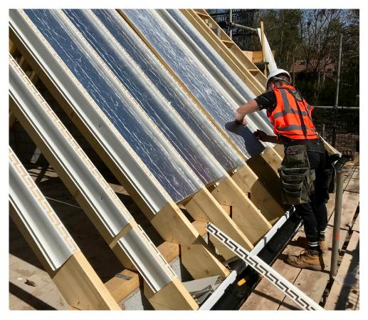
"I came up with the idea of a Track that simply fits over the rafter with a retaining ledge that locks the board into place." alongside current energy prices, the payback time on using the Insulfix solution is only about 3.7 years.
